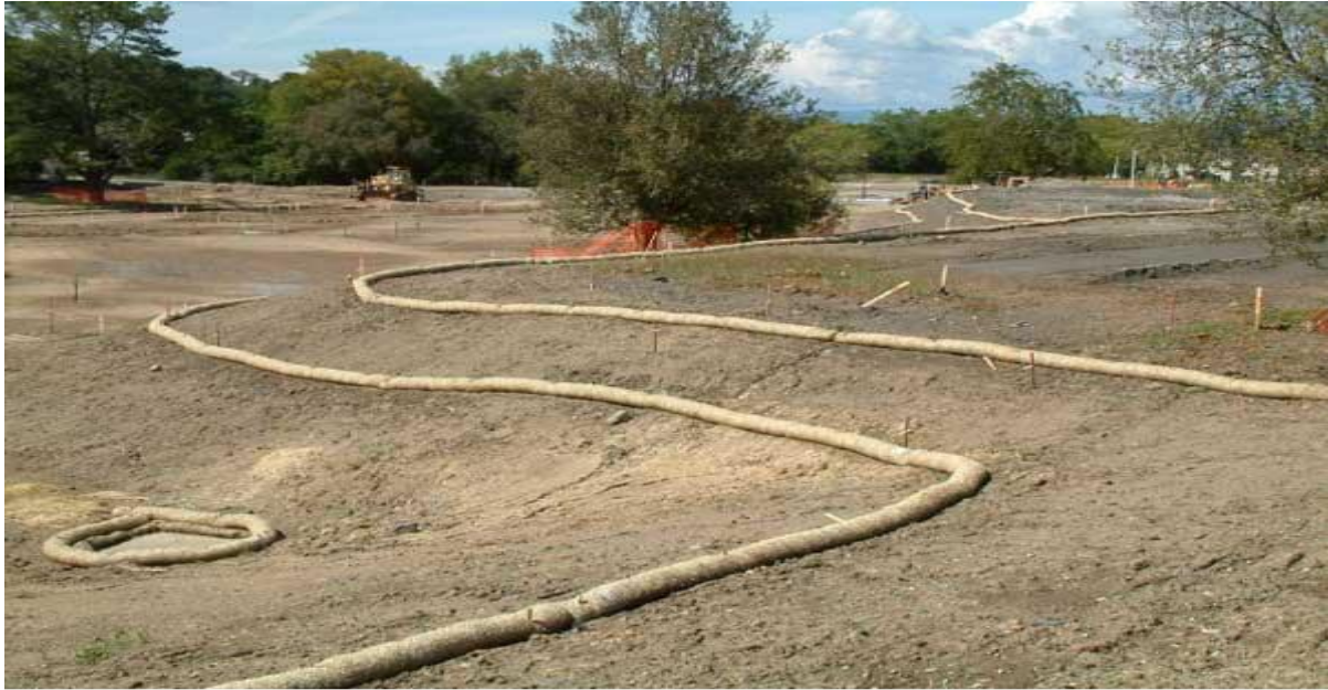
Figure 48: Erosion control in cultivated land using wattle construction
