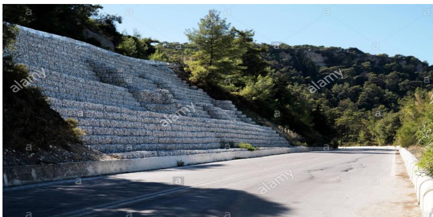
Figure 45: Gabions for protecting road destruction
