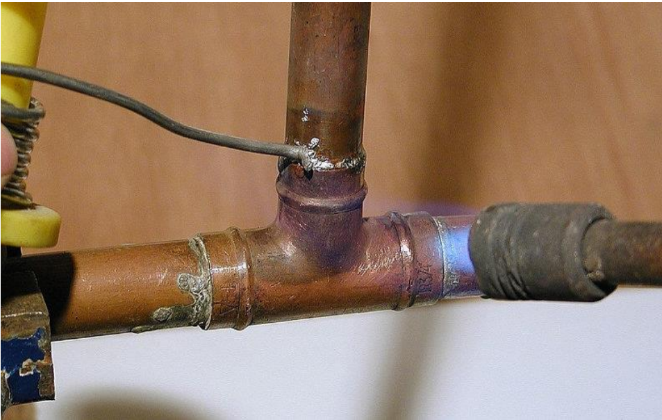
Figure: Capillary joint
