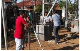
Fig.6: Checking Verticality Using Theodolite
