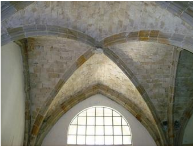
Cross-ribbed vault, Bonne-Espérance Abbey, Vellereille-les-Brayeux, Belgium, ca, 13th century: Ogival, or pointed arches, increased in popularity in the Gothic period.
