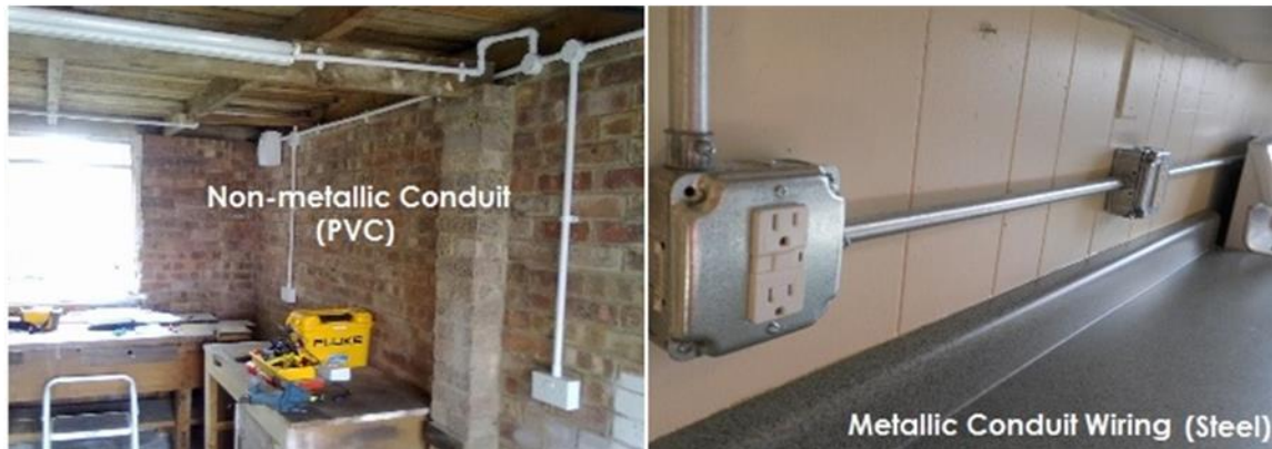
Figure 1.Surface mounted
