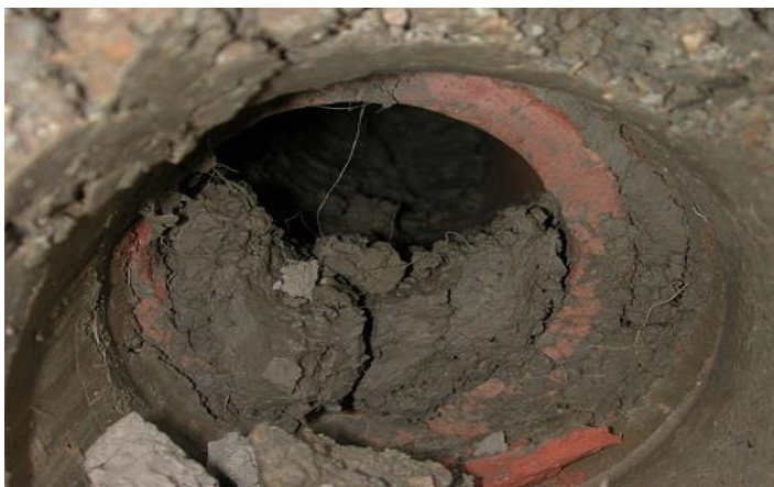
Figure: Drain pipe containing a significant amount of sediment
