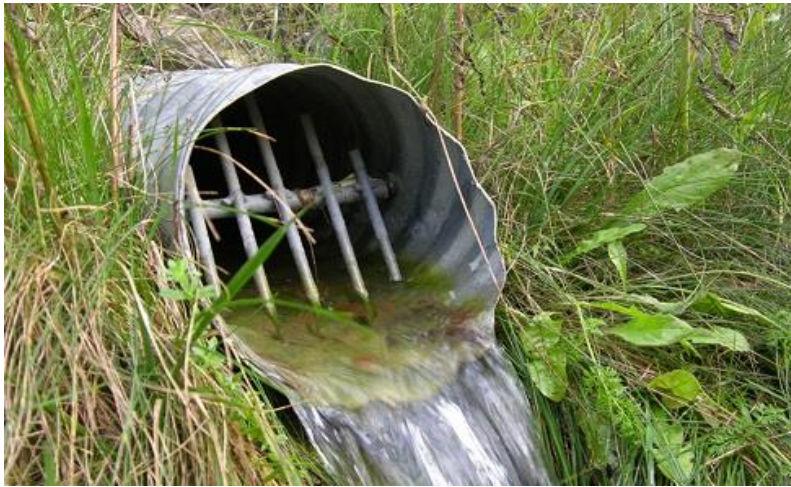
Figure: Outfall pipe with rodent guard installed
