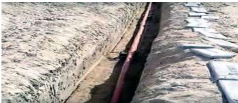
**Draw in system** cable layout methods is widely used for heavily populated areas such as urban cities and towns. Normally the cables are layout in ducts or pipelines on the ground with certain holes.
