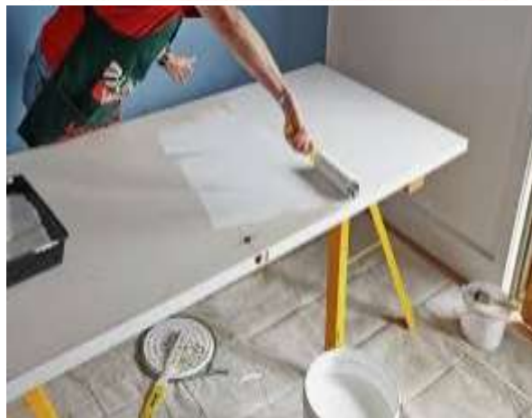
Figure 13: Applying anti corrosion coating product
