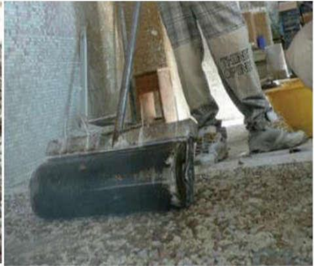
compacting exposed marble chips with compactor roller
